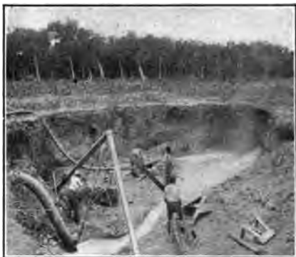
FIG. 111. — Hydraulic mining of phosphate rock in Florida.
